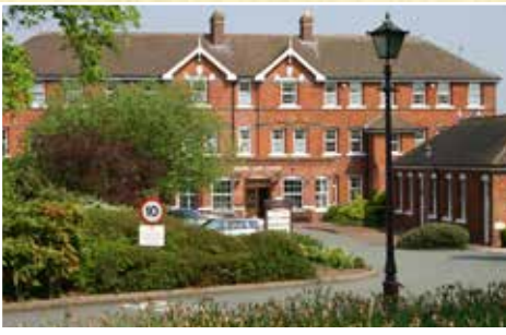
Wellington Workhouse Infirmary: its inmates were sent to Wolverhampton between 1916 and 1919, when nearly 3,000 wounded soldiers were treated there.
