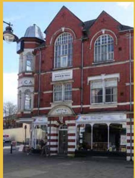
The Wrekin Hall: situated on the top floor of the Wrekin Buildings in Walker Street.
